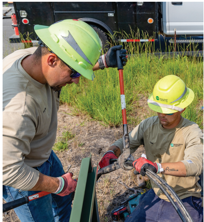
Teamwork is key as Kyle Childers and Evan Mizzell work together to set an underground service in Hewing Farms subdivision in Summerville.
