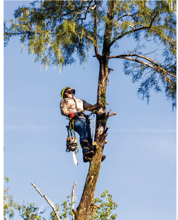
Line Clearance Foreman Jeremy Walker removes a tree endangering a power line to prevent a future outage.
